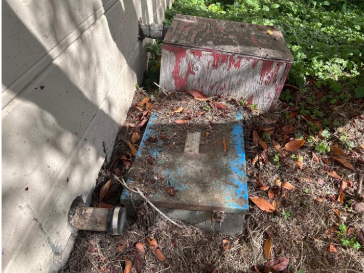
EXTERIOR EAST WALL- GREASE TRAP
