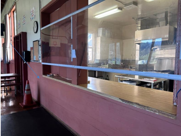
NORTH WALL FACING GYM – ARROW FOR HYDRATION STATION
