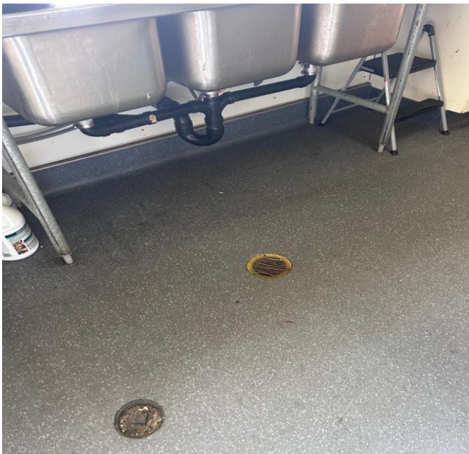
EAST WALL FLOOR
