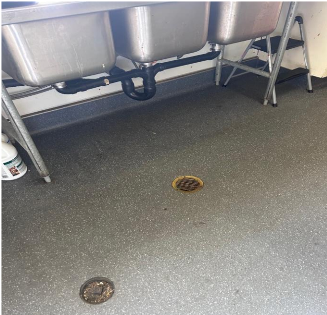
EAST WALL FLOOR
